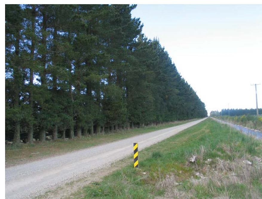
Looking along Dixon Road towards east
