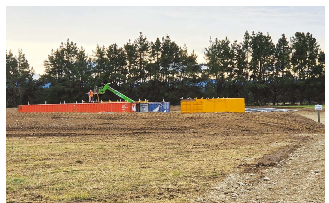
Site office preparation works.
