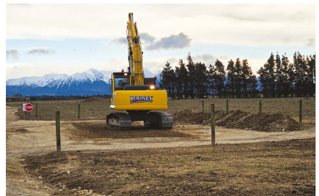
Site preparation works for the diesel fuel storage facility.
