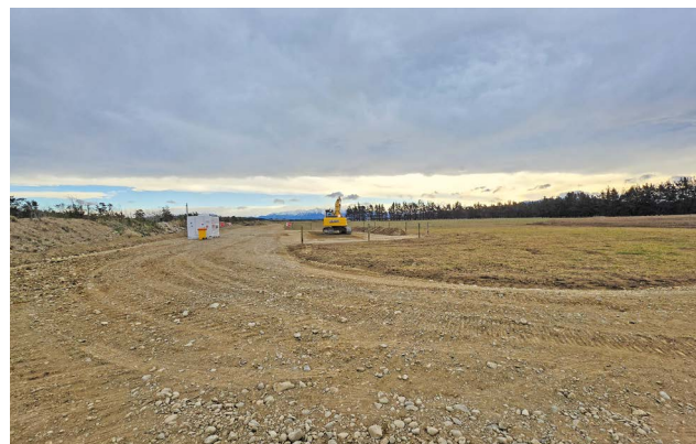
Site preparation works for the diesel storage facility with access road to the storage ponds construction site in the background.
